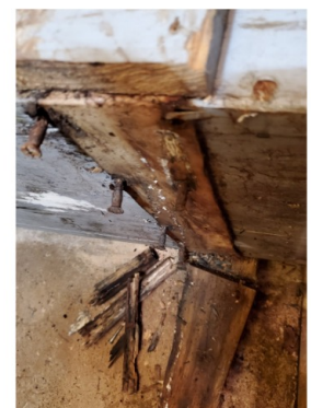
Pictured above, old wiring that was replaced, and water damage caused by flooding in 2018.
