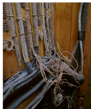
Pictured above, old wiring that was replaced, and water damage caused by flooding in 2018.
